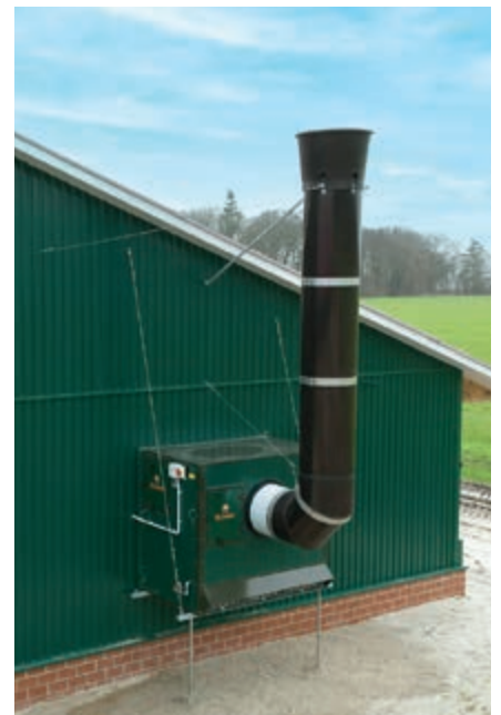
Earny2 S installed at the gable
