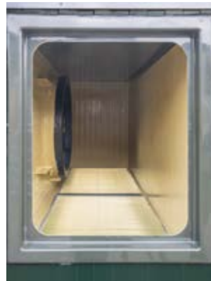
View into Earny2 S: the fan pulls the warmed fresh air into the house
