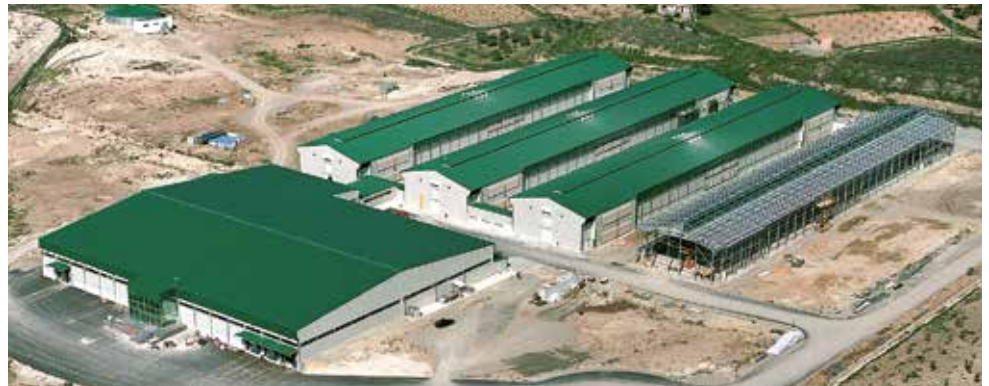
Farm Grupo Avícola la Cresta in Bullas, Spain, for a total of 1 million laying hens
