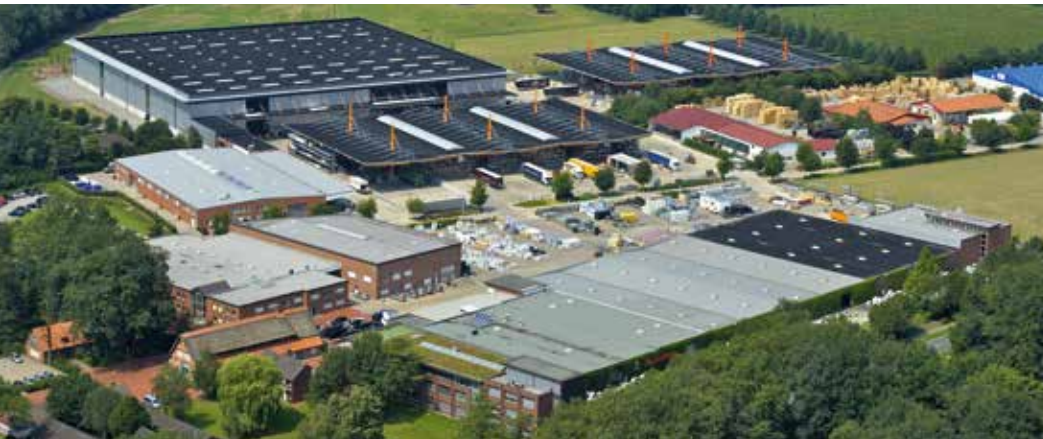
Big Dutchman headquarters in Vechta, Germany
