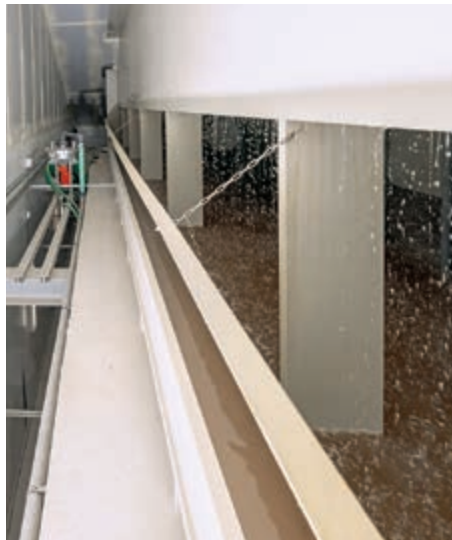
An exhaust air cleaner is used to clean the ammonia from the OptiSec Porco exhaust air
